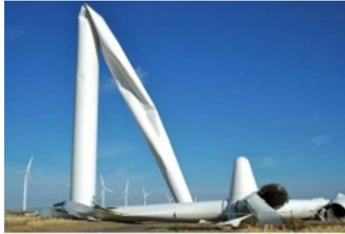
Figure 4. Large scale wind turbine failure due to buckling.
